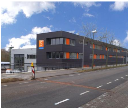
View from Saarbrücker Strasse
