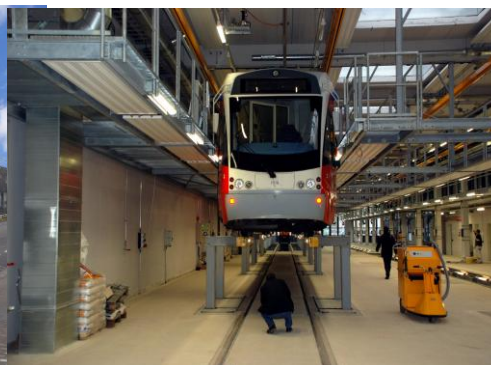
Workshop hoist for under floor inspection
