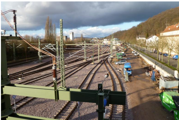
New stabling yard and track leading into the workshop (Source: WGK)
