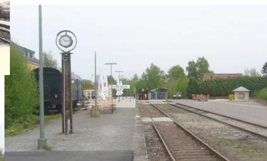
Kranenburg, rail-cycle draine station
